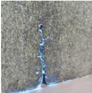
Photograph shows a crack in a block wall before the seam tape is applied.
