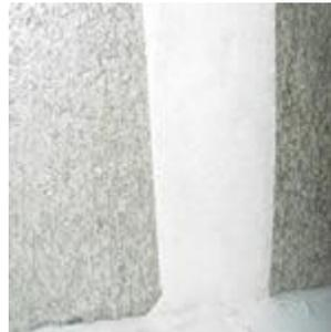
Crack is sealed with the shaping seam tape and coated with Ames' Block & Wall elastomeric rubber coating.
